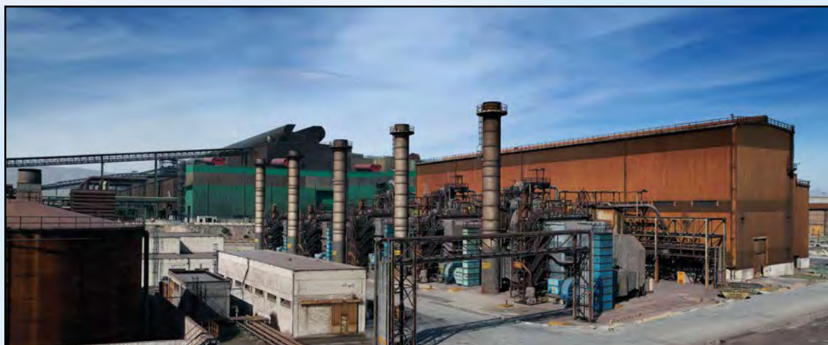
1- Integrated Iron and Steel Mill
